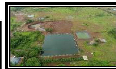
Rainwater harvesting structures to utilise rainwater for industrial processes
