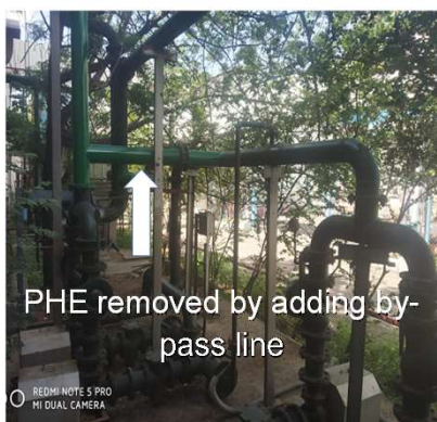
Picture after modification
